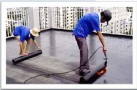
Waterproofing torch membrane
