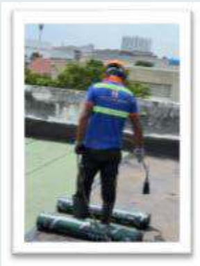
Torch bitumen membrane
