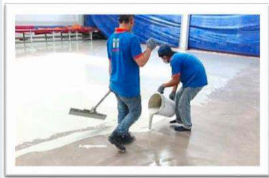
DHL TSN AIRPORT SELF LEVELING EPOXY 3MM
