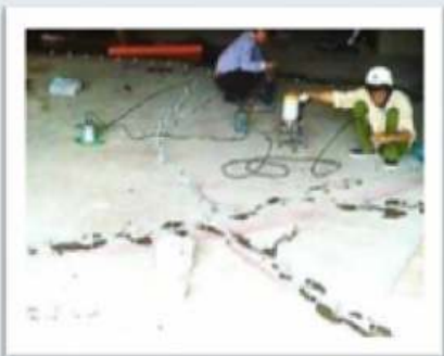
Welding the CONCRETE crack
