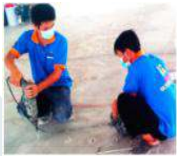
EPOXY PUMP TO WELD CONCRETE CRACKS
