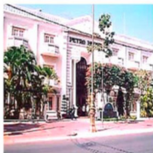
PETRO HOUSE (VUNG TAU)
