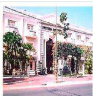
PETRO HOUSE (VUNG TAU)
