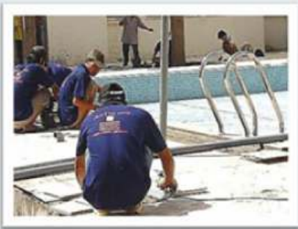
Construction of the pool
